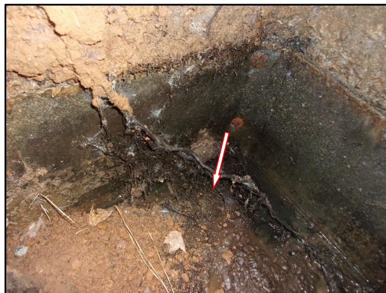
Extensive Root Infiltration:
