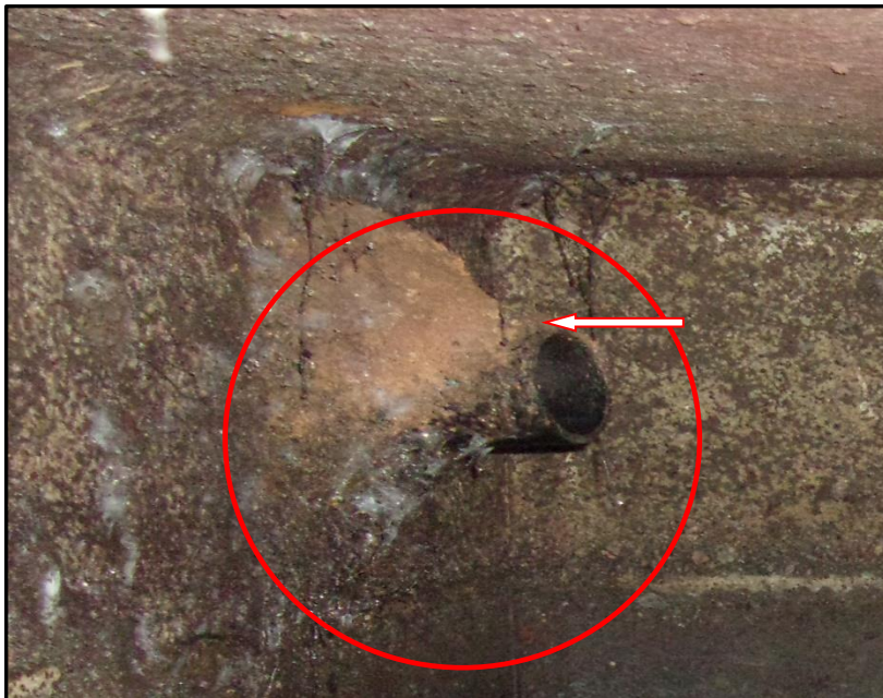
Outlet Wastewater Supply Pipe (Root Infiltration):
