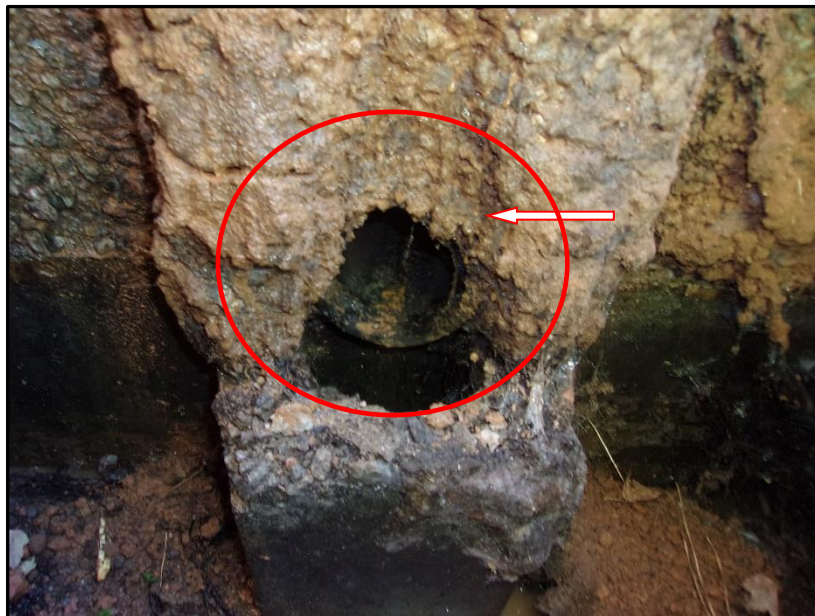
Outlet Wastewater Supply Pipe (Root Infiltration):
