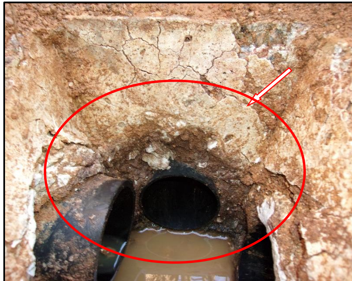
Broken and Deteriorated Lid:
