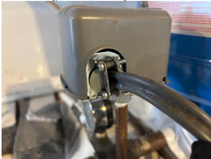
Pressure storage tank contact relay shown sealed
