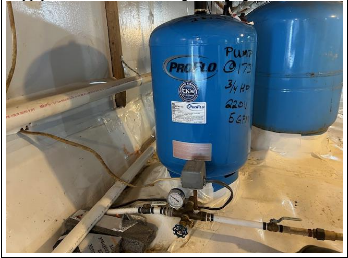
Supply line shown terminating through ground
