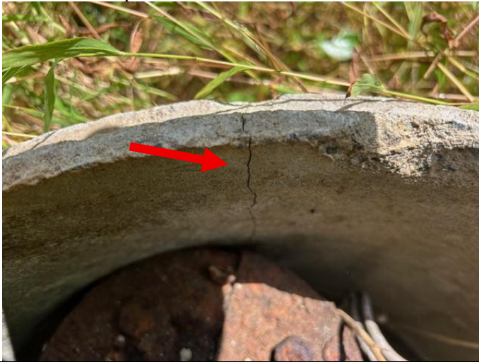
Crack on well protective cover
