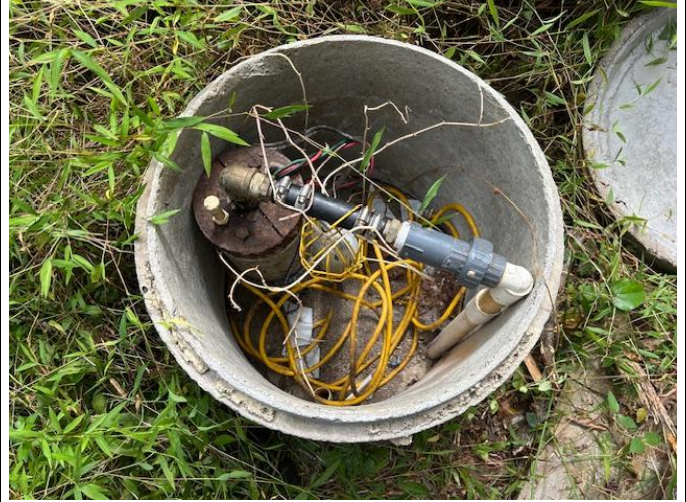
Electrical wires shown not properly sealed in junction box
