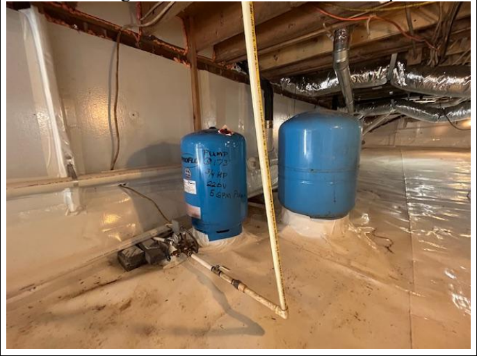
Pressure storage tank location shown in crawlspace
