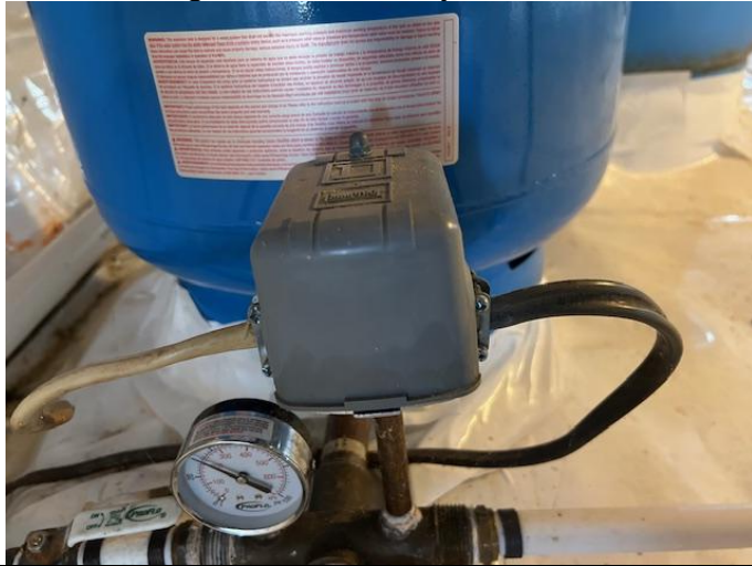
Pressure storage tank contact relay shown sealed
