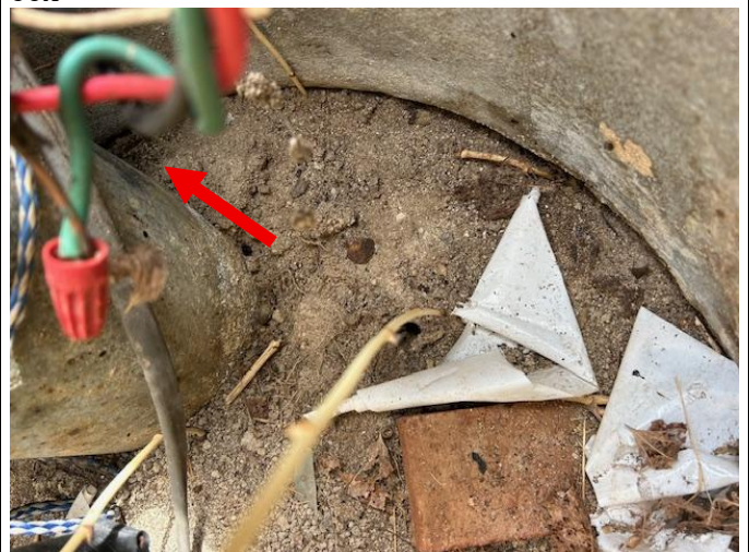
Electrical wires shown not properly sealed in junction box
