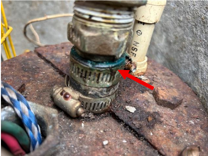
Crack on well protective cover
