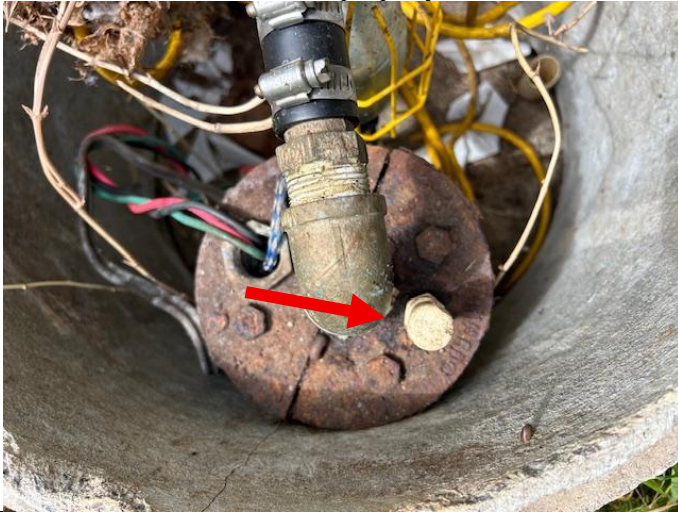
Leak noted at well head
