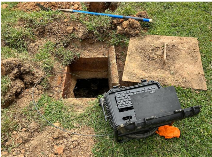
Outlet line shown scoped.
