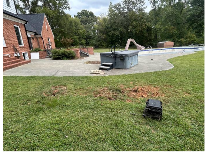
Septic tank location shown covered up post-inspection.
