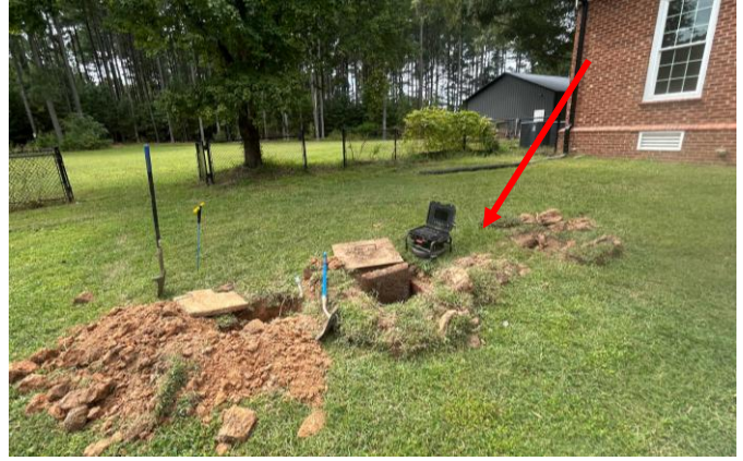
Inlet riser shown less than 3" above grade.
