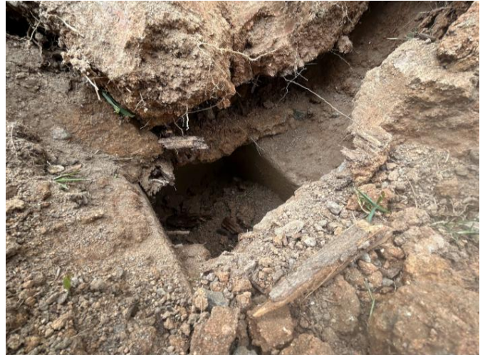
Inlet riser shown less than 3" above grade.
