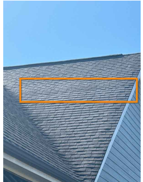
Front Right Roof
