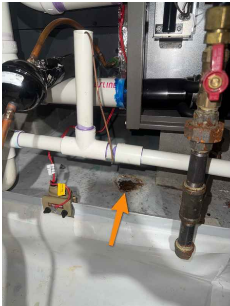
Crawlspace Middle Rear
