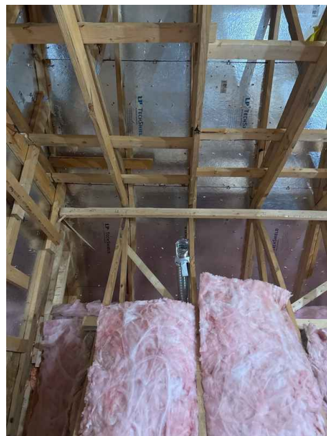
2nd Floor Bathroom
