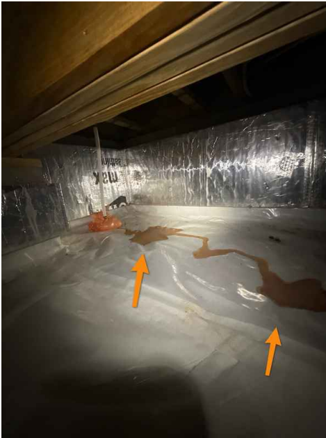
Front Right Crawlspace
