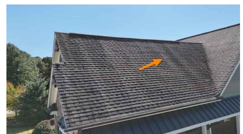
Front Right, Garage
