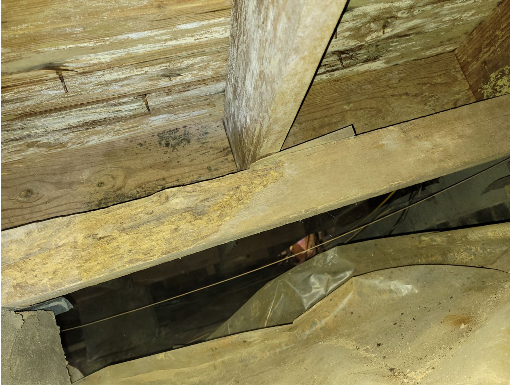
Moisture damaged wall framing
