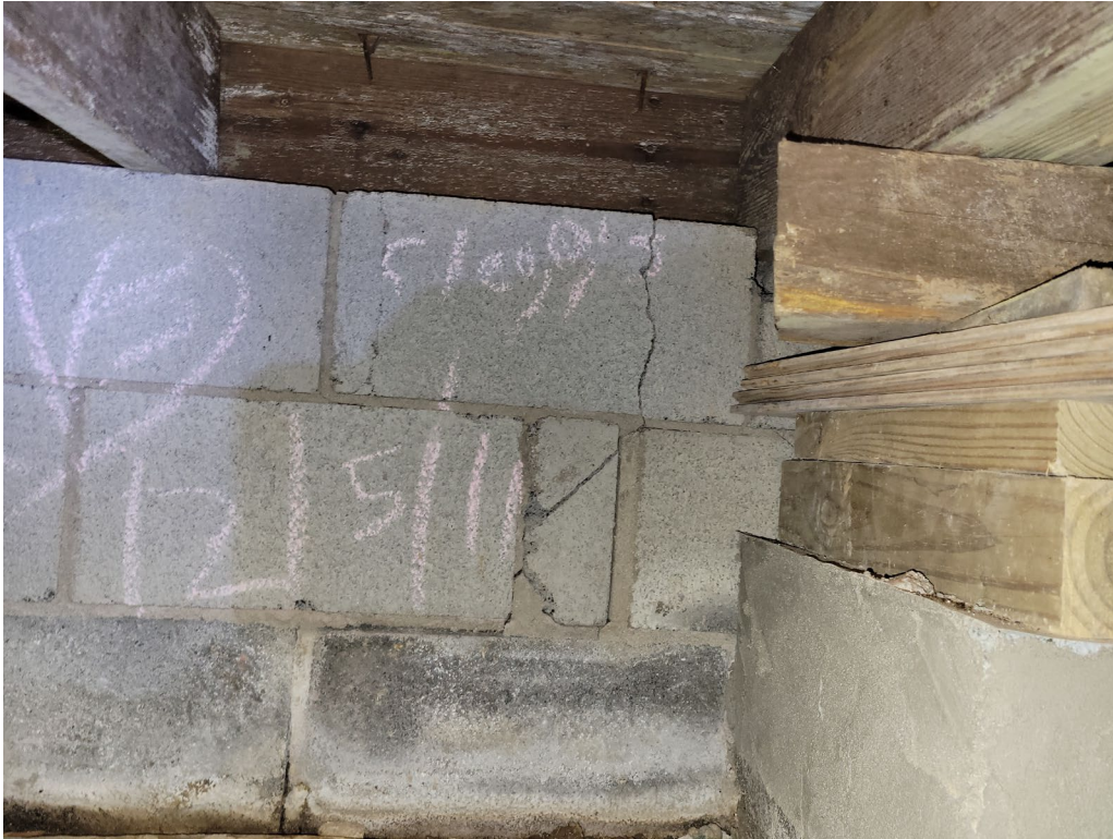
Foundation Crack:
