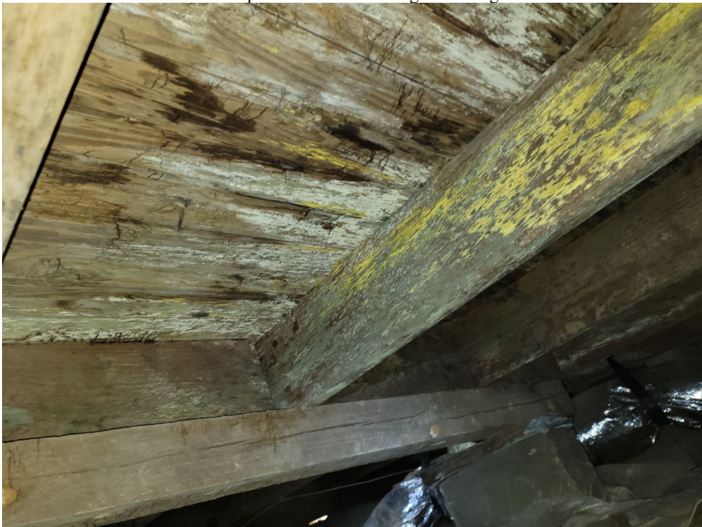
Examples of moisture damaged framing:
