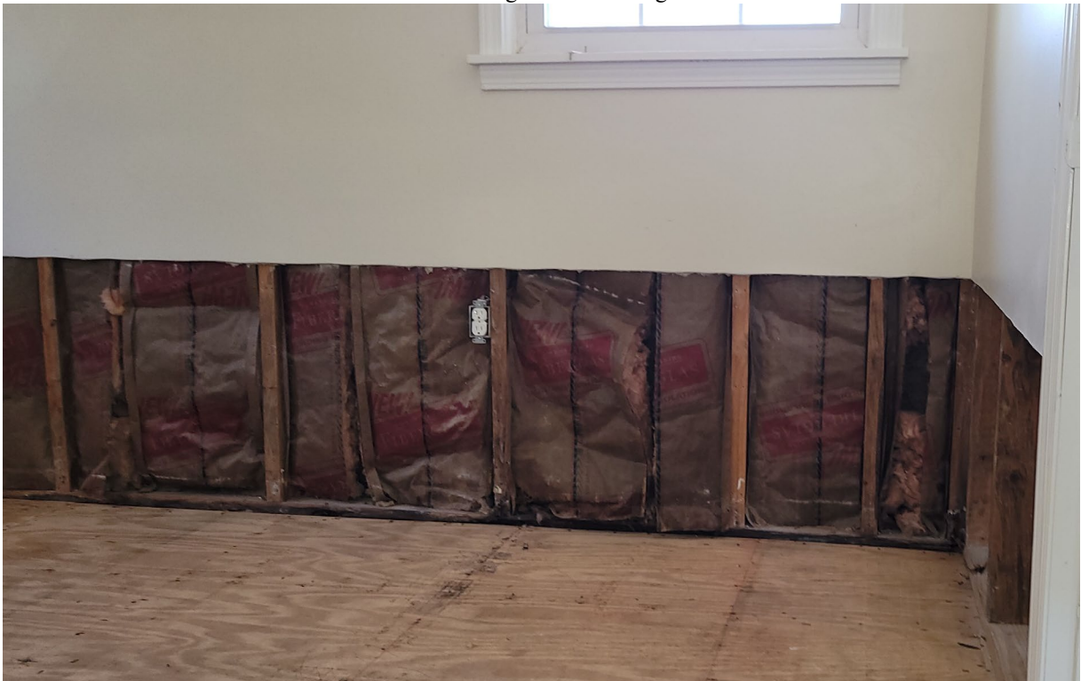
Moisture damaged wall framing
