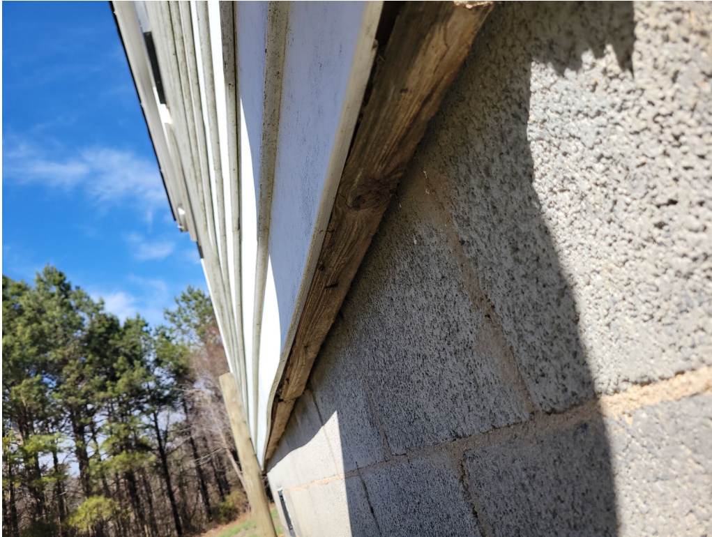
Front band shifted off foundation wall:
