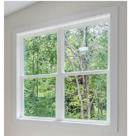
Window Casing: 90* angle
