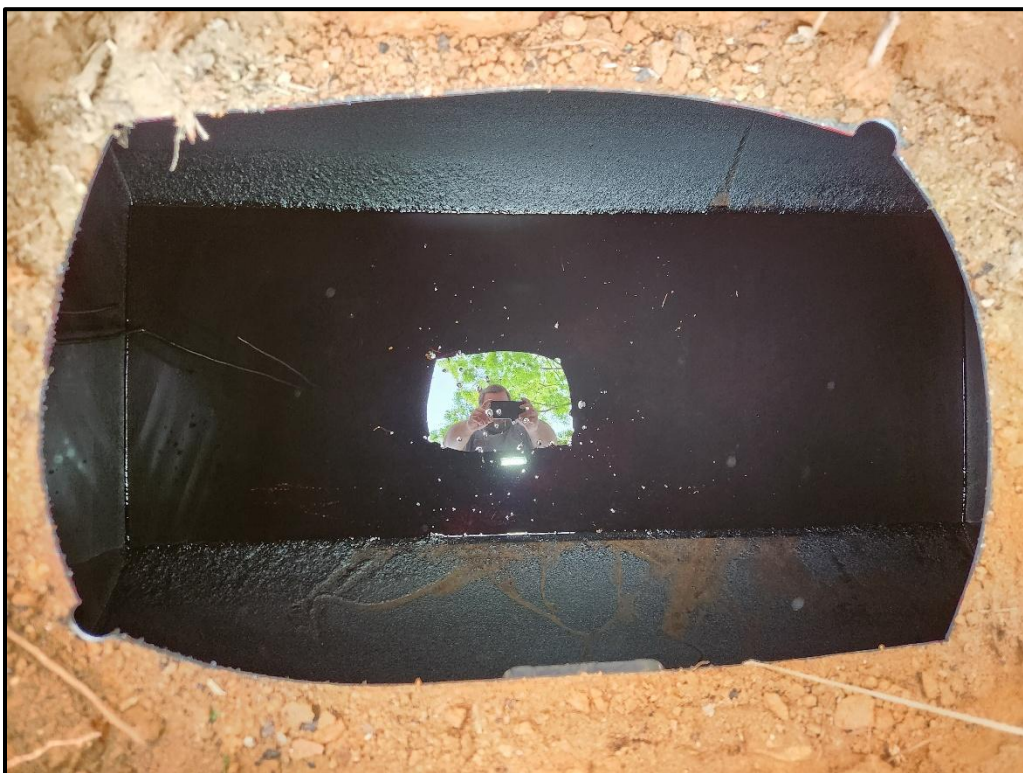
Photo 2. View of the UST interior prior to the removal of tank contents.
