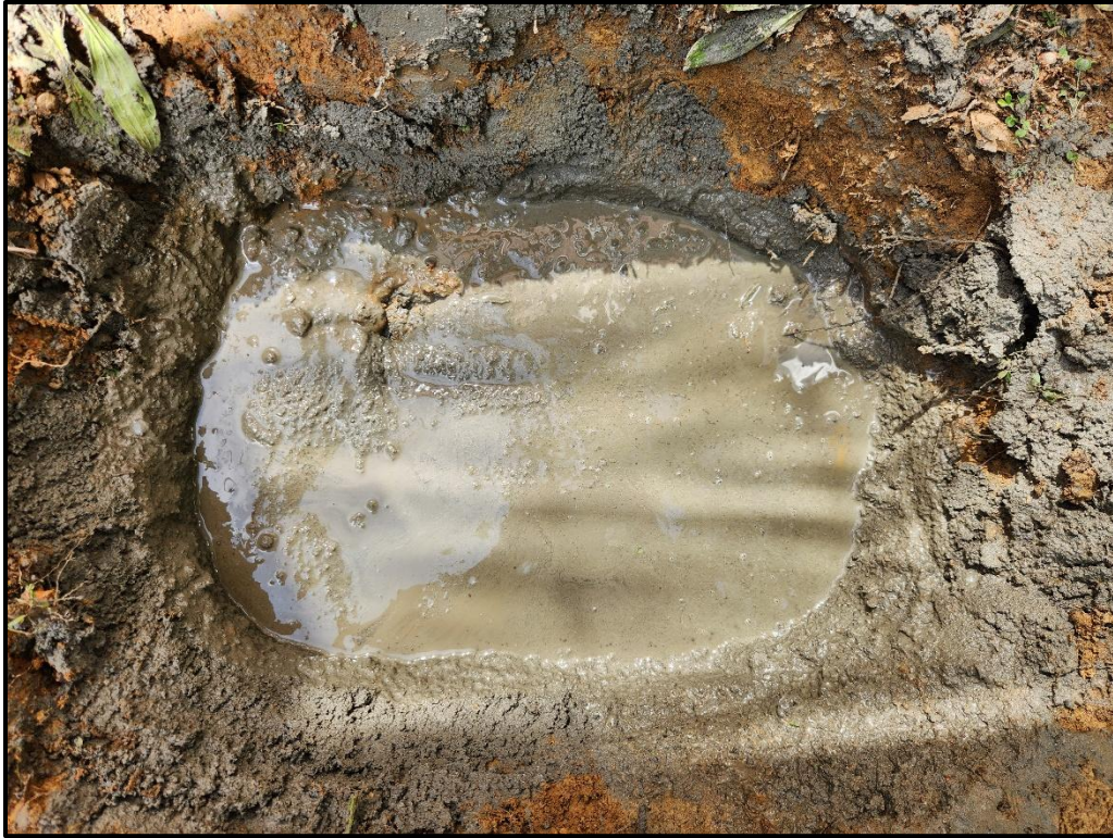
Photo 5. View of the UST after filling with flowable fill cement slurry.
