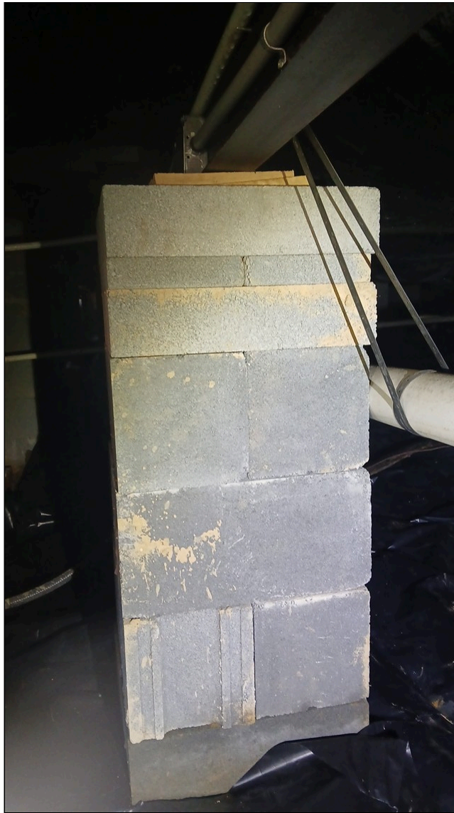
11.0 FOUNDATION WALLS/ PIERS / COLUMNS / FLOOR FRAMING / MAIN BEAM(S) (Picture 1)
