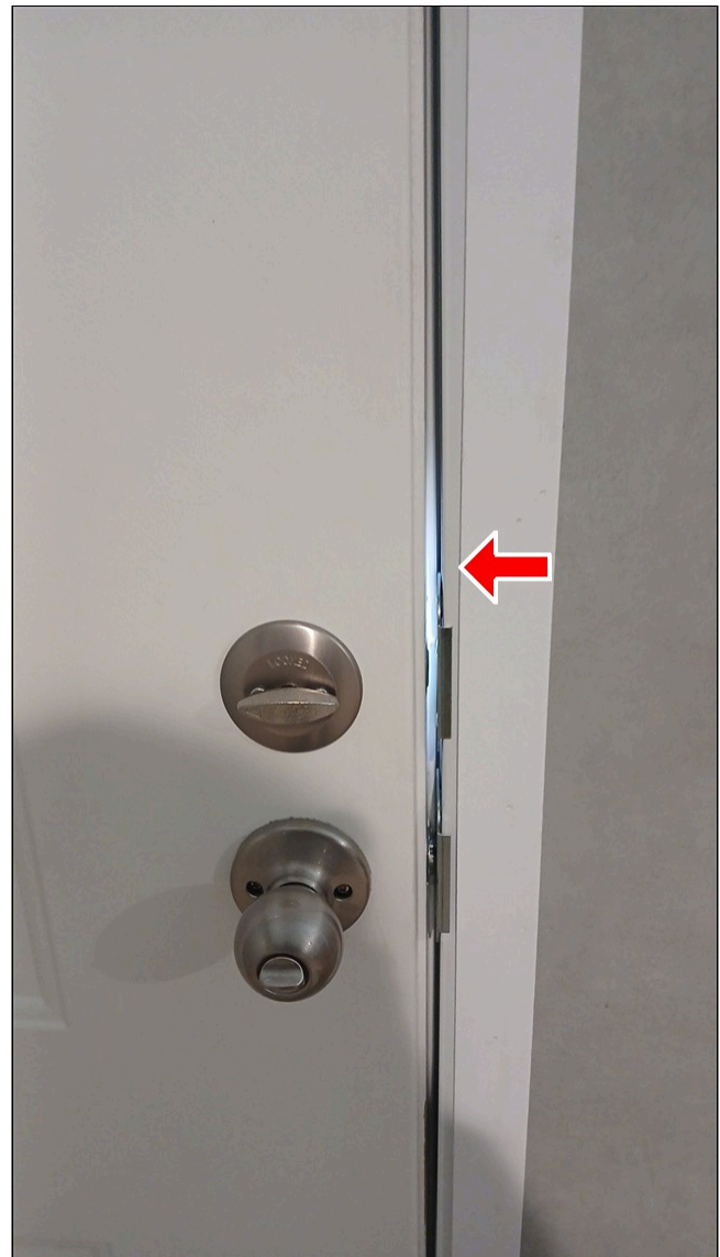
2.2(1) ENTRY DOORS (Picture 2)
