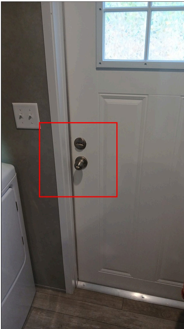
2.2(2) ENTRY DOORS (Picture 1)
