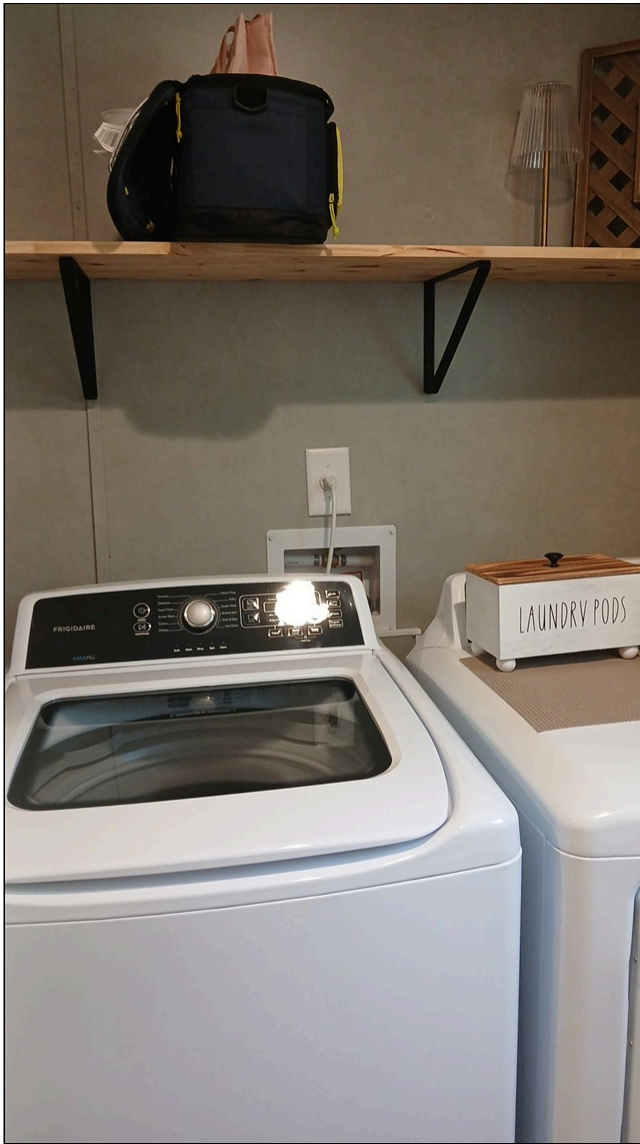
9.0 MAIN WATER CUTOFF (Picture 1)
