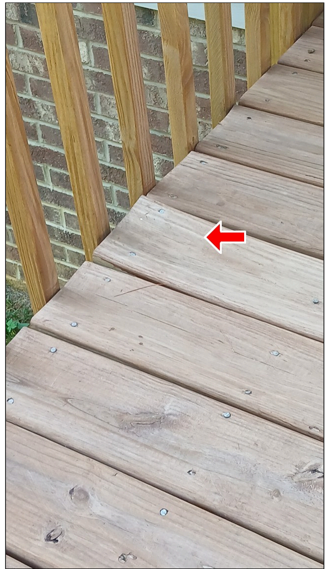
2.3 STAIRS / STOOPS / RAILINGS (Picture 2)
