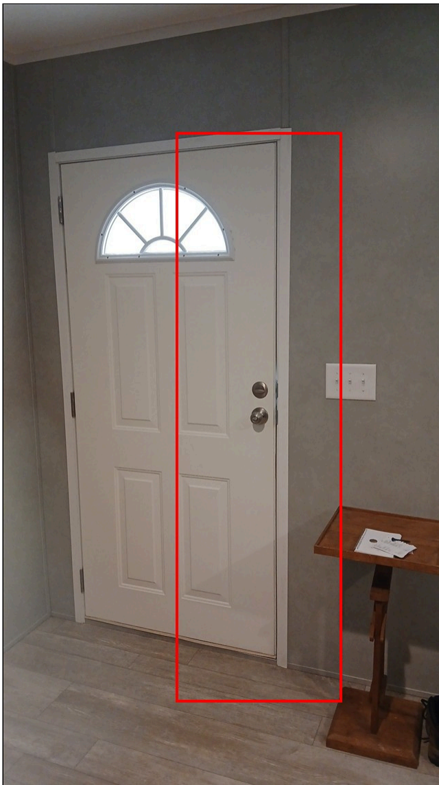
2.2(1) ENTRY DOORS (Picture 1)
