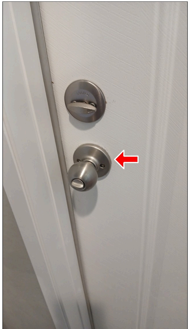
2.2(2) ENTRY DOORS (Picture 2)
