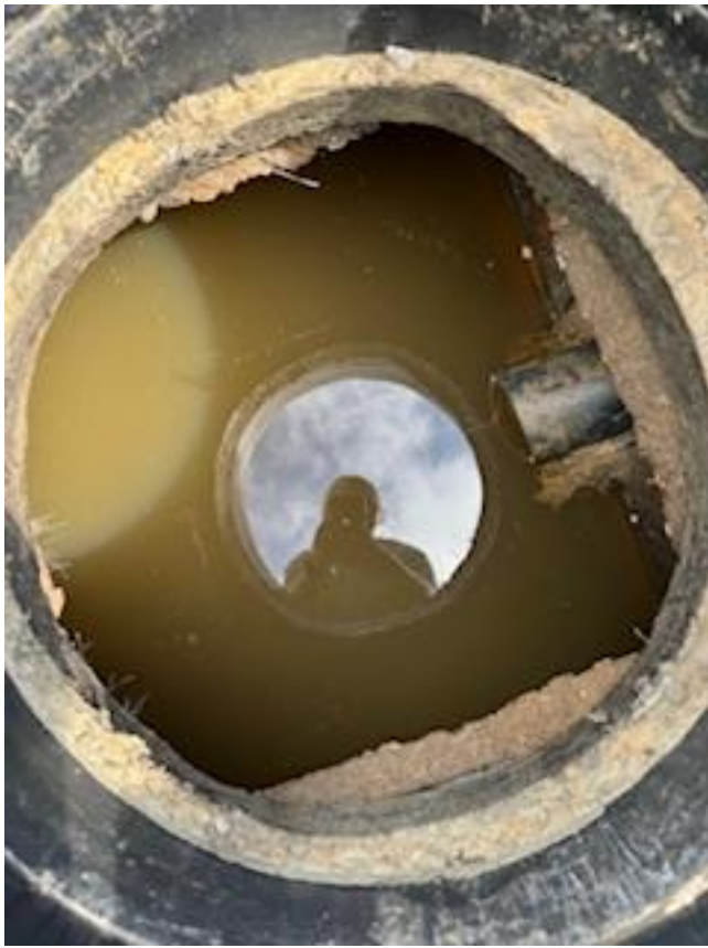
INLET OF TANK
