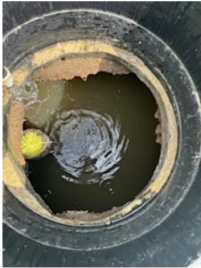
OUTLET OF TANK
