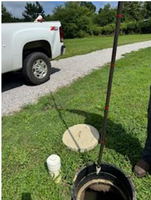
OUTLET SLUDGE MEASURE and CLEANOUT
