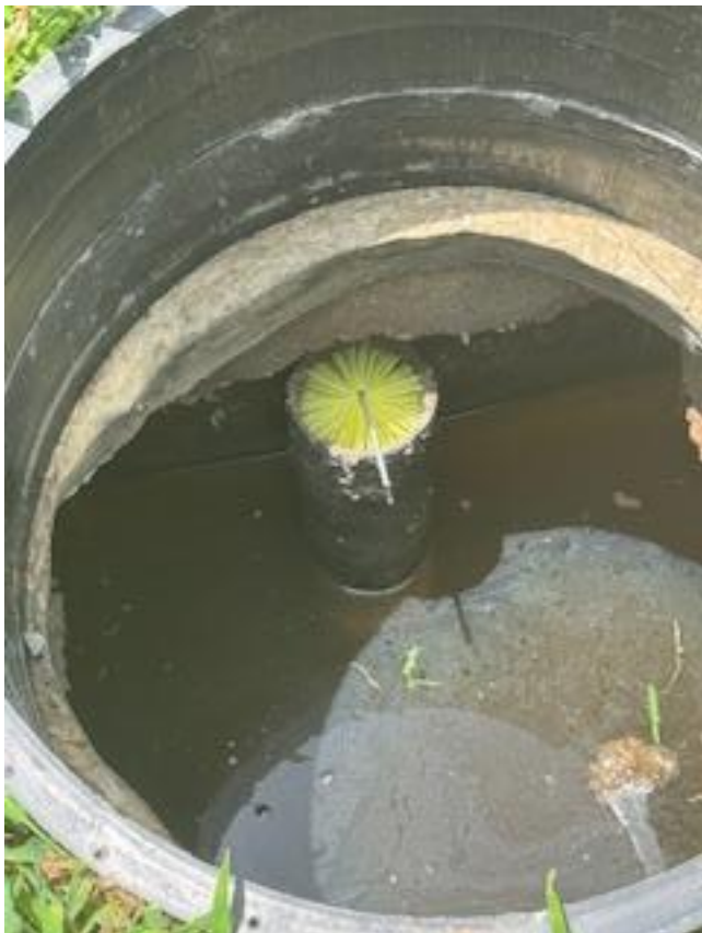
TANK TEE and FILTER – OUTLET
