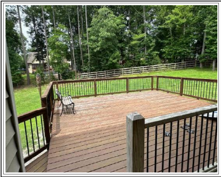
Rear wood deck
