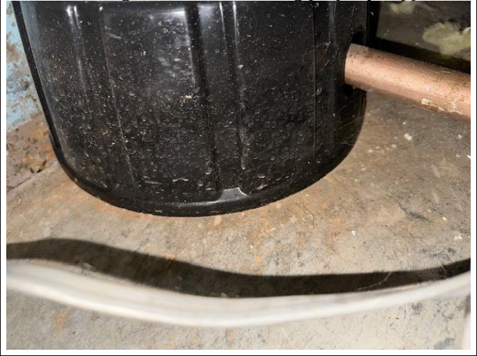
Signs of leaks at the sediment filter
