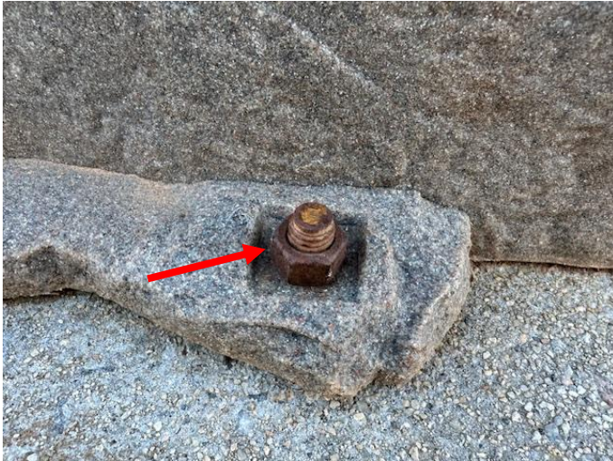
Bolts and nuts noted as corroded not removed
