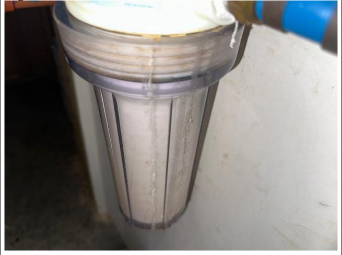
Signs of leaks at the sediment filter
