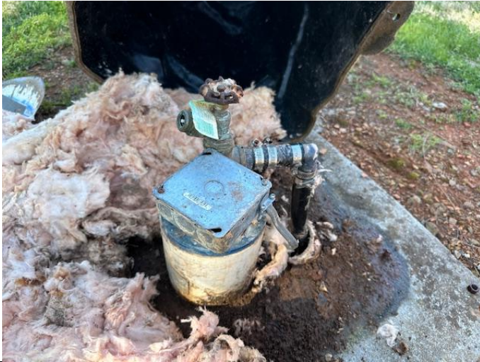
Well head casing seal shown
