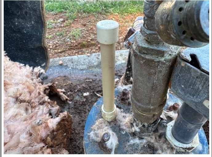
Fittings shown properly sealed (no leaks)
