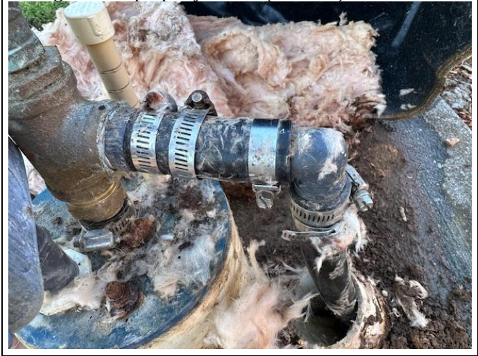
Fittings shown properly sealed (no leaks)
