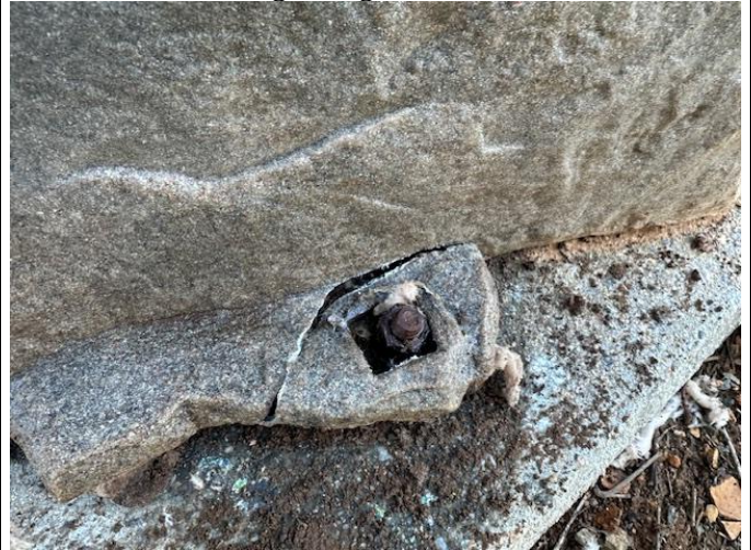
Insulated rock damaged to gain access to well head
