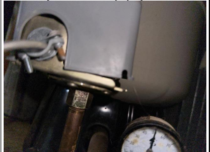
Contact relay cover shown not properly sealed
