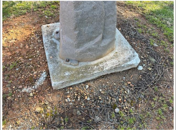
Insulated rock damaged to gain access to well head
