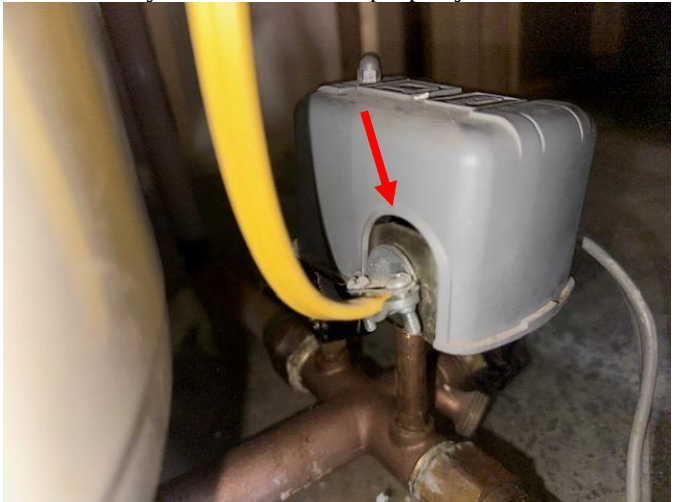
Contact relay cover shown not properly sealed
