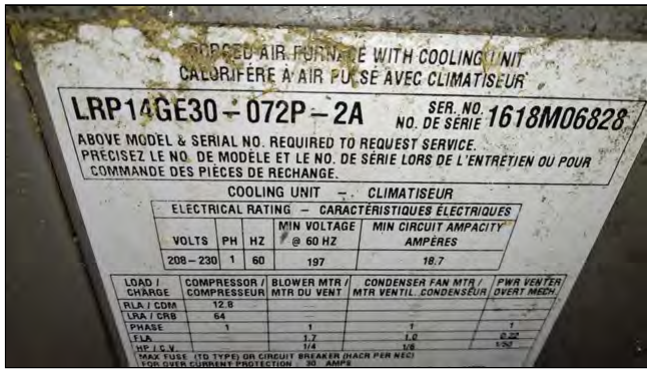
10.1 Item 1(Picture) The package unit Mfg label
