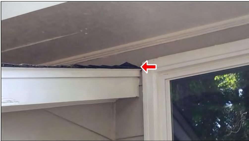
3.0 Item 1(Picture) Lifter shingle over the flashing on he rear storage room
