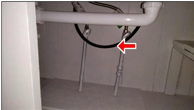
12.6 Item 1(Picture) Missing sprayers weight
