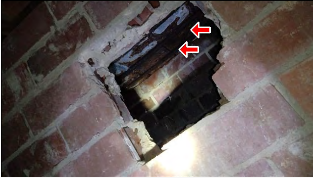
2.5 Item 1(Picture) Heavy rust damage to the front porch support metal
