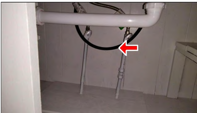
12.6 Item 1(Picture) Missing sprayers weight
