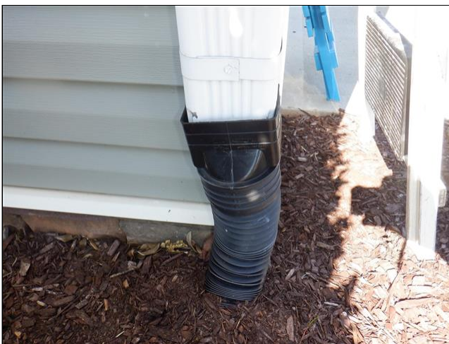
1.3(1) RAIN GUTTERS / EAVETROUGHES / DOWNSPOUTS / ROOF DRAINS (Picture 1) front and rear sides
