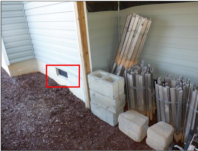
13.0(1) FOUNDATION WALLS/ PIERS / COLUMNS / FLOOR FRAMING / MAIN BEAM(S) (Picture 5)
