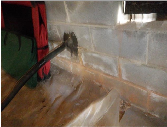
13.0(2) FOUNDATION WALLS/ PIERS / COLUMNS / FLOOR FRAMING / MAIN BEAM(S) (Picture 2)
