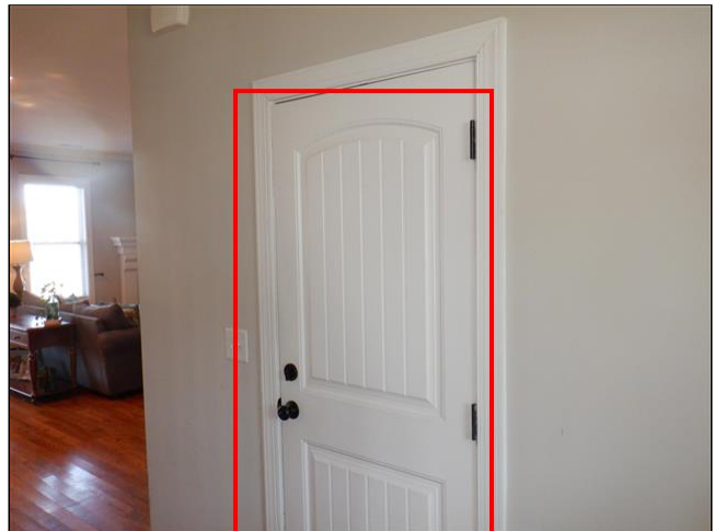
2.4(1) ENTRY DOORS (Picture 1)
