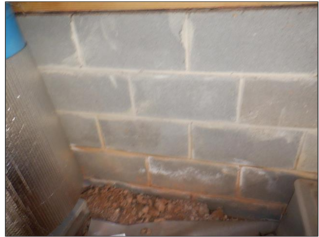
13.0(2) FOUNDATION WALLS/ PIERS / COLUMNS / FLOOR FRAMING / MAIN BEAM(S) (Picture 1)
