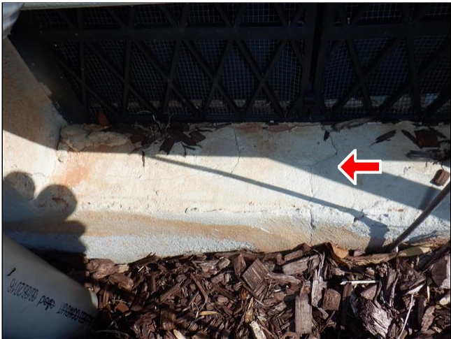
13.0(1) FOUNDATION WALLS/ PIERS / COLUMNS / FLOOR FRAMING / MAIN BEAM(S) (Picture 2)
