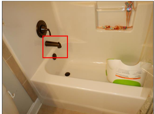
8.1(1) BATHTUB (Picture 1) upper level hall bathtub
