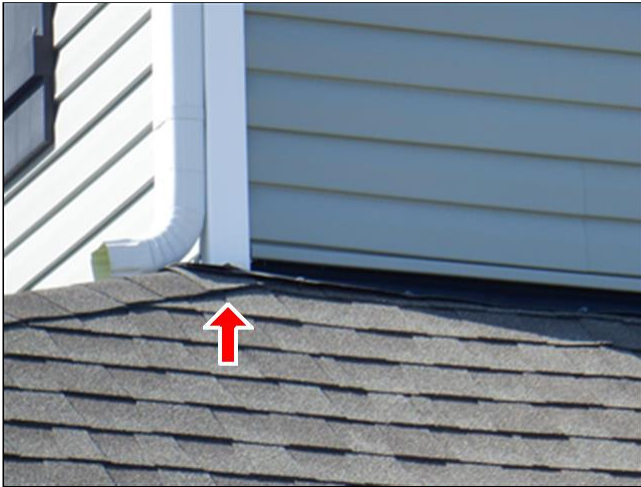
1.2 EXPOSED FLASHING (s) (Picture 2)
