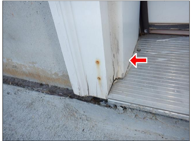
2.4(3) ENTRY DOORS (Picture 3)
