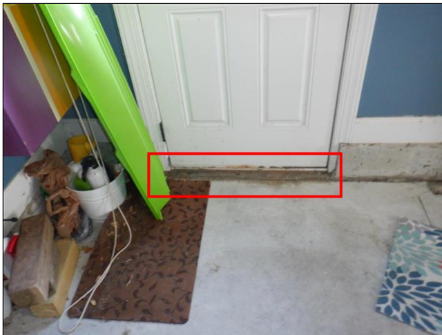
2.4 (4) Cracked mortar at garage door. Recommend caulk/seal due to water intrusion concerns.
