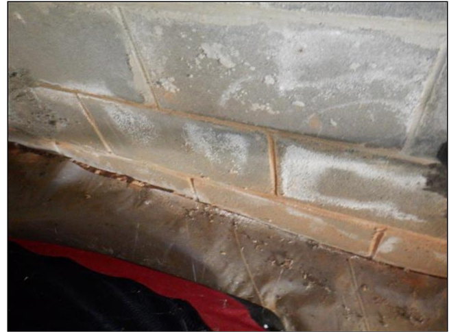
13.0(2) FOUNDATION WALLS/ PIERS / COLUMNS / FLOOR FRAMING / MAIN BEAM(S) (Picture 3)
