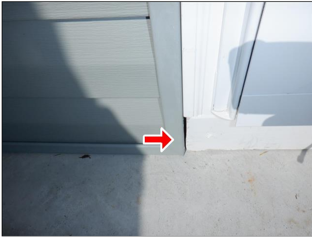
2.4(2) ENTRY DOORS (Picture 3)
