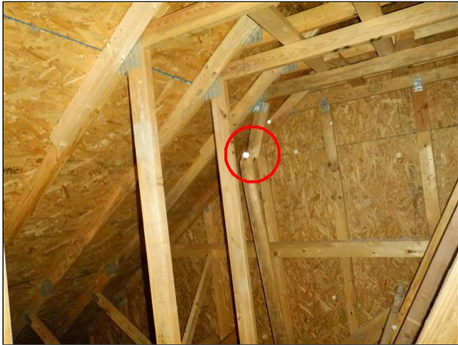
5.0 ROOF FRAMING (Picture 1)
