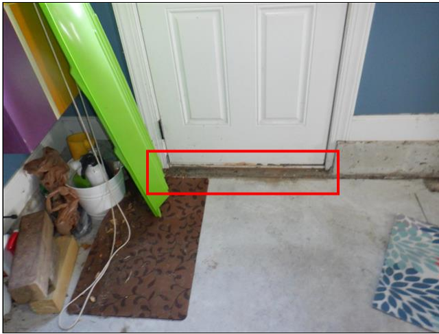
2.4(4) ENTRY DOORS (Picture 1)
