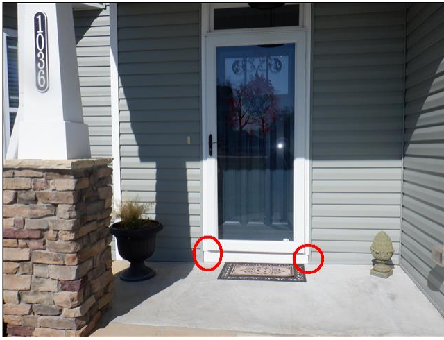
2.4(2) ENTRY DOORS (Picture 1)
