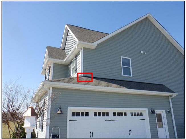
1.2 EXPOSED FLASHING (s) (Picture 1)
