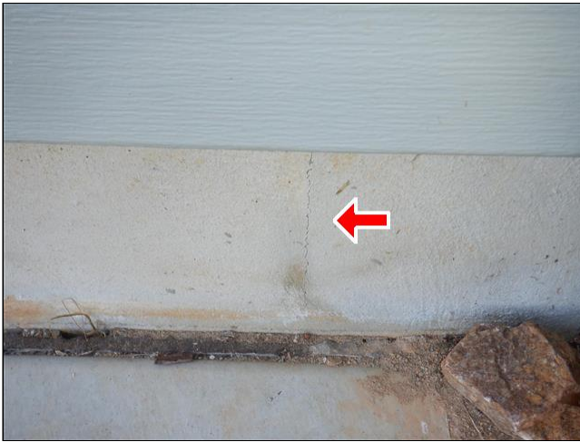
13.0(1) FOUNDATION WALLS/ PIERS / COLUMNS / FLOOR FRAMING / MAIN BEAM(S) (Picture 11)
