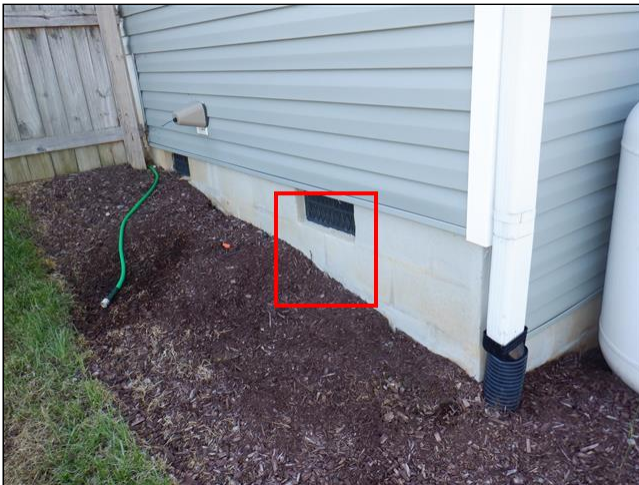
13.0(1) FOUNDATION WALLS/ PIERS / COLUMNS / FLOOR FRAMING / MAIN BEAM(S) (Picture 7)
