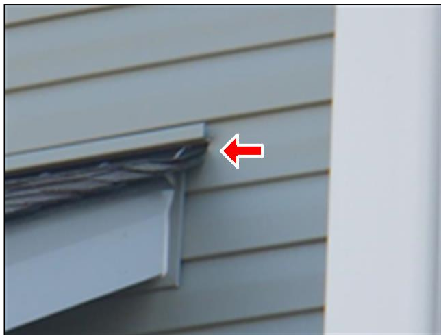
1.2 EXPOSED FLASHING (s) (Picture 4)
