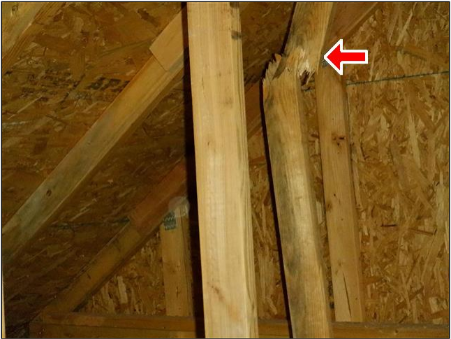
5.0 ROOF FRAMING (Picture 2)
