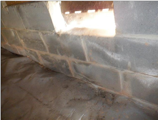
13.0(2) FOUNDATION WALLS/ PIERS / COLUMNS / FLOOR FRAMING / MAIN BEAM(S) (Picture 4)
