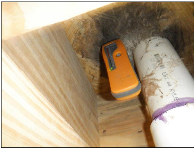
13.0(3) FOUNDATION WALLS/ PIERS / COLUMNS / FLOOR FRAMING / MAIN BEAM(S) (Picture 2)
