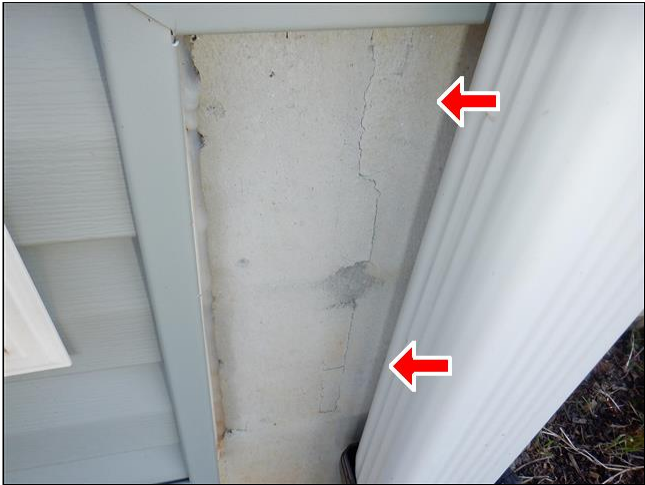
13.0(1) FOUNDATION WALLS/ PIERS / COLUMNS / FLOOR FRAMING / MAIN BEAM(S) (Picture 4)
