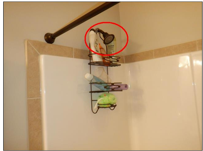
8.1(2) BATHTUB (Picture 1) upper level hall bathtub
