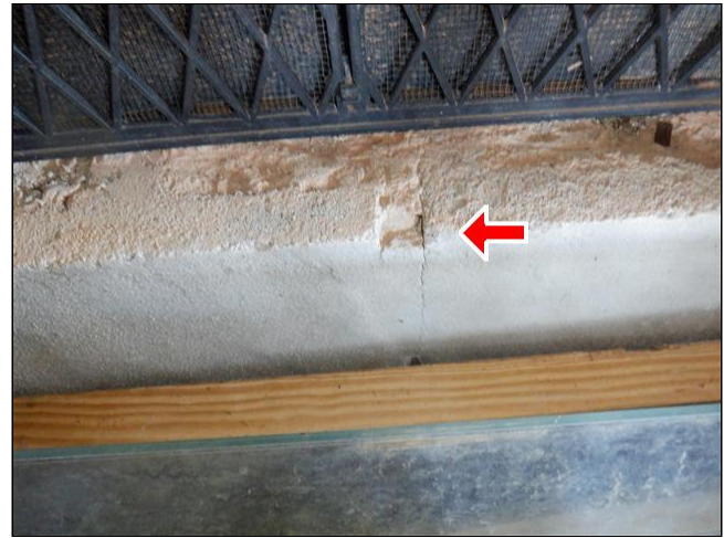
13.0(1) FOUNDATION WALLS/ PIERS / COLUMNS / FLOOR FRAMING / MAIN BEAM(S) (Picture 6)
