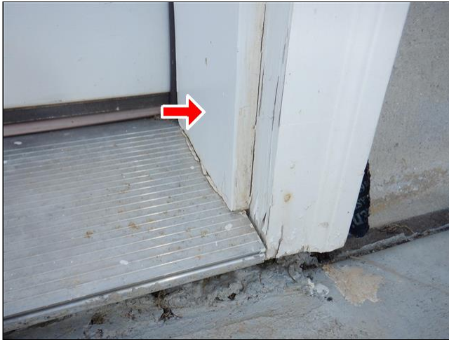
2.4(3) ENTRY DOORS (Picture 2)
