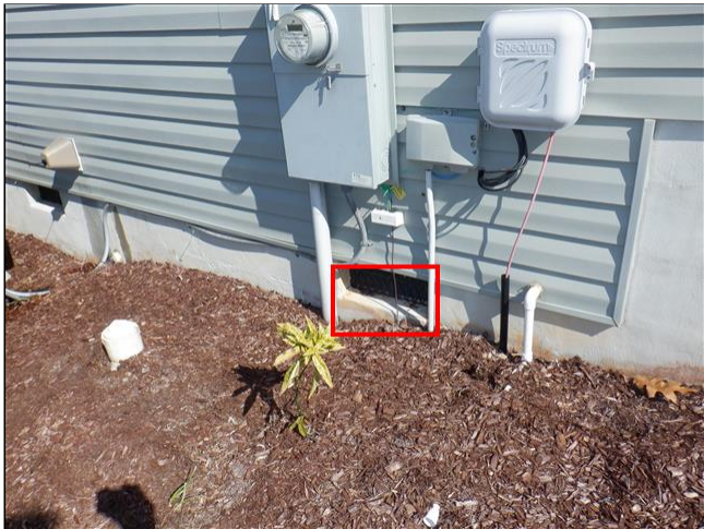
13.0(1) FOUNDATION WALLS/ PIERS / COLUMNS / FLOOR FRAMING / MAIN BEAM(S) (Picture 1)
