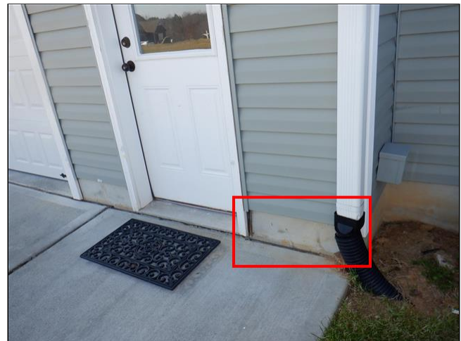
13.0(1) FOUNDATION WALLS/ PIERS / COLUMNS / FLOOR FRAMING / MAIN BEAM(S) (Picture 10)
