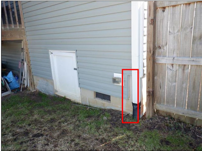
13.0(1) FOUNDATION WALLS/ PIERS / COLUMNS / FLOOR FRAMING / MAIN BEAM(S) (Picture 3)
