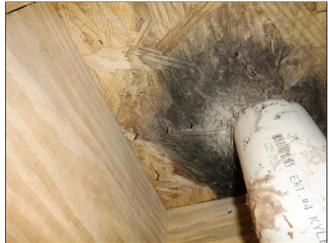
13.0(3) FOUNDATION WALLS/ PIERS / COLUMNS / FLOOR FRAMING / MAIN BEAM(S) (Picture 1)
