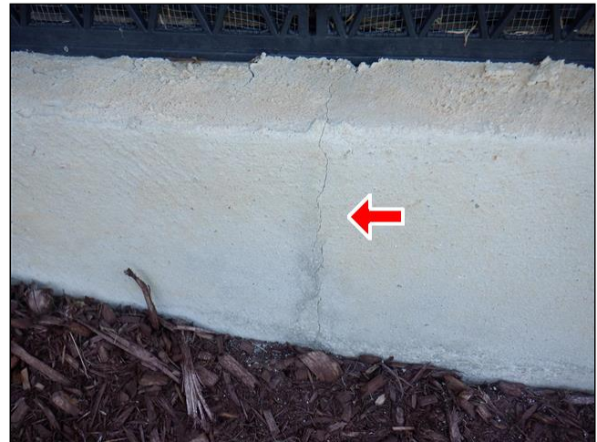
13.0(1) FOUNDATION WALLS/ PIERS / COLUMNS / FLOOR FRAMING / MAIN BEAM(S) (Picture 8)
