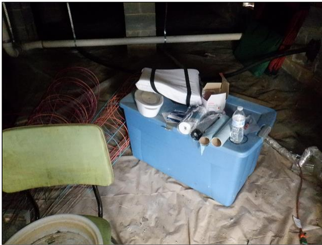
13.4 CRAWLSPACE DEBRIS/CELLULOSE (Picture 2)
