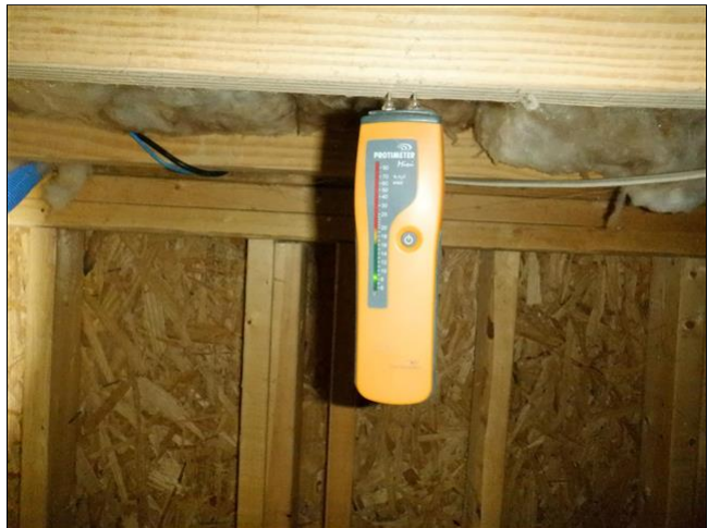
right rear 9% moisture
