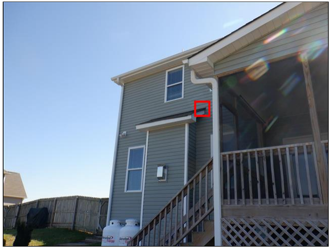
1.2 EXPOSED FLASHING (s) (Picture 3)
