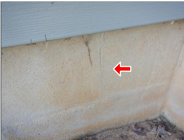
13.0(1) FOUNDATION WALLS/ PIERS / COLUMNS / FLOOR FRAMING / MAIN BEAM(S) (Picture 9)
