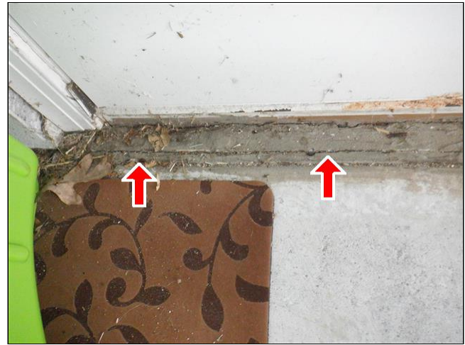
2.4(4) ENTRY DOORS (Picture 2)
