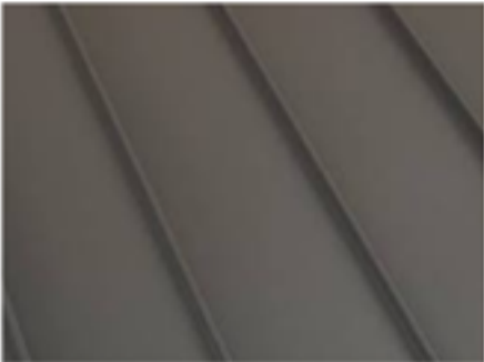
Dark Bronze Metal Porch Roof and Gutters
