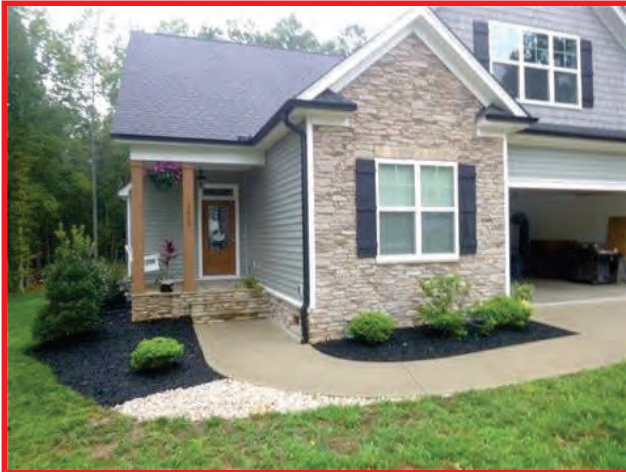
Missing Handrails at Front Steps
