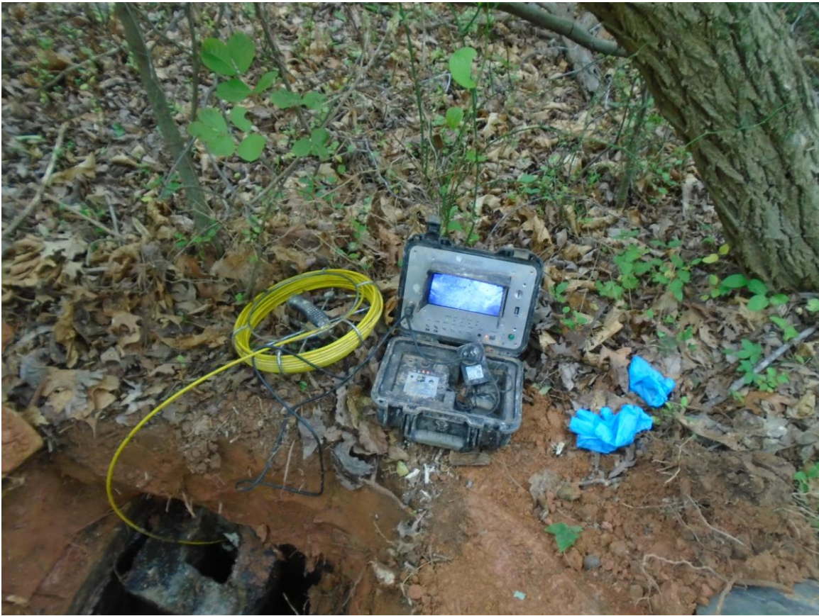
Camera Inspection of Drainfield Line
