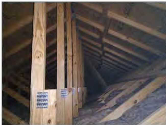
1.1 Item 1(Picture) The roof framing
