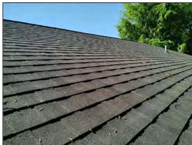
2.0 Item 1(Picture) The shingles appear to be original from 2017
