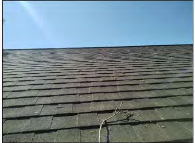
2.0 Item 2(Picture) Shingles appears to be original
