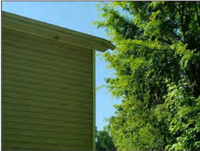
2.1 Item 1(Picture) Damaged gutters
