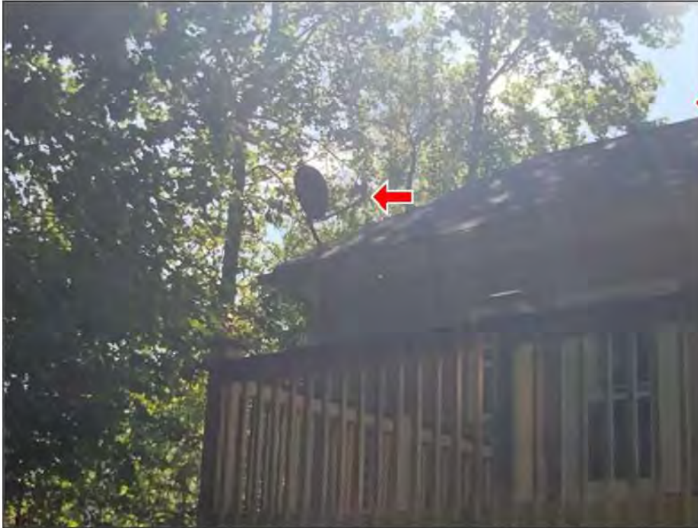
2.0 Item 4(Picture) Satellite frame in place on the roof coverings
