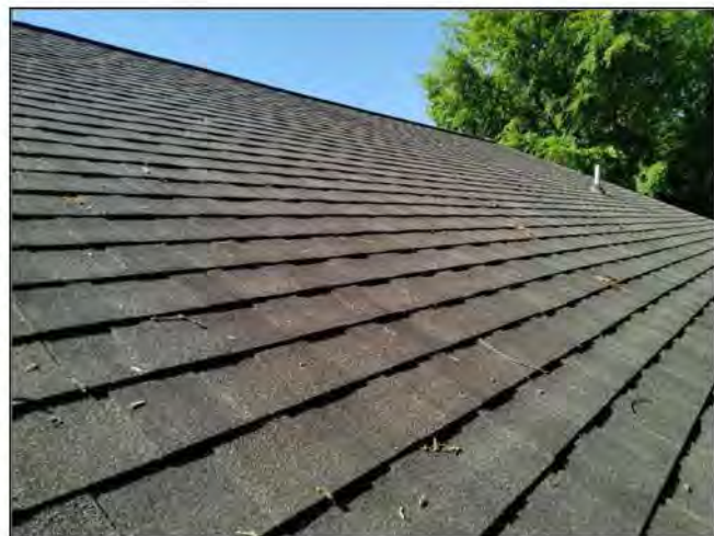
2.0 Item 3(Picture) Shingles appears to be original
