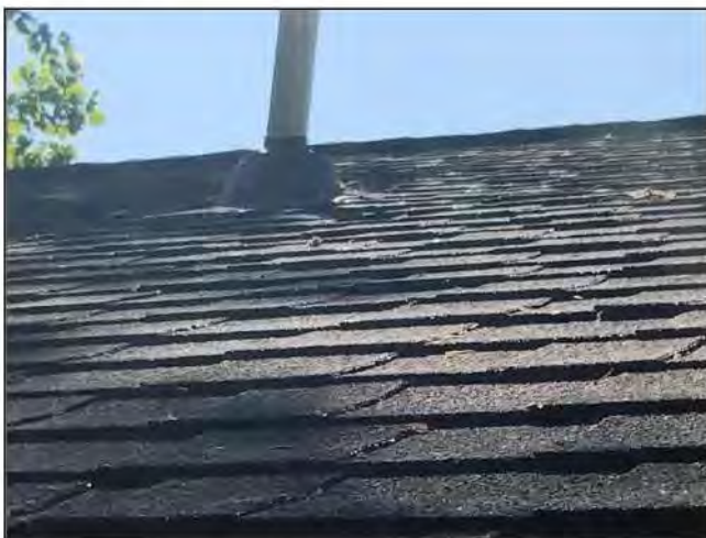
2.2 Item 1(Picture) Plumbing boots look to be functional with no signs of leaks
