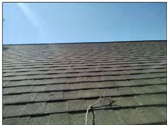
2.0 Item 2(Picture) Shingles appears to be original
