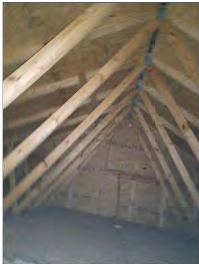
1.1 Item 2(Picture) The roof framing
