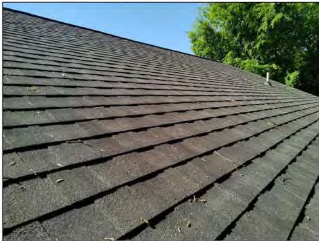
2.0 Item 3(Picture) Shingles appears to be original
