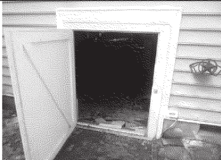
Crawl Space Entry at Rear
