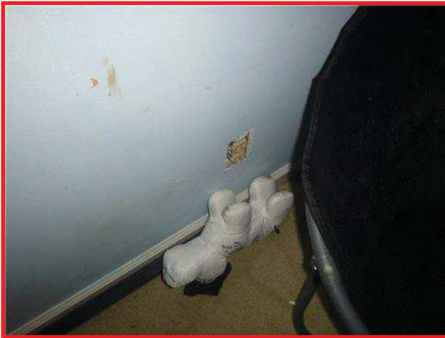
Missing Outlet Cover
