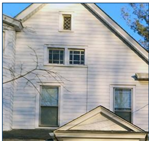
The vinyl siding has covered the dwelling's historic architectural features, including original siding, trim, and fascia. The pediment seen in the bottom part of the photograph shows what original materials would have been visible – scalloped shingles and detailed fascia.
