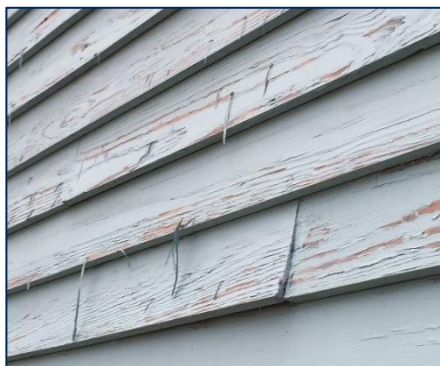
Example of a wood surface in need of repainting. Gentle handscraping would likely be sufficient for preparing the surface for new paint.
