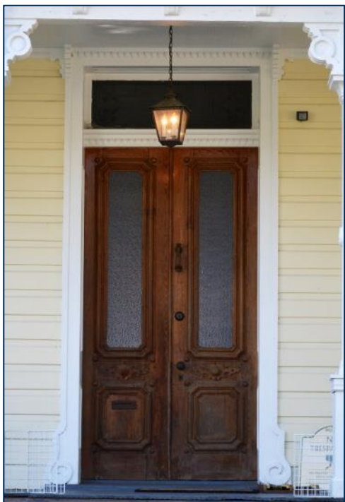
Historically appropriate lantern-style porch light fixture
