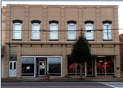
This rehabilitated storefront features the large windows, recessed doorways, and dropped cornice that so often characterize historic storefronts.
