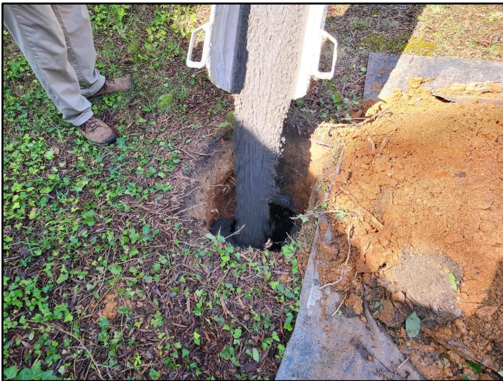
Photo 4. View of the UST being filled with flowable fill cement slurry.
