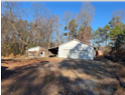
Exterior building was not inspected
