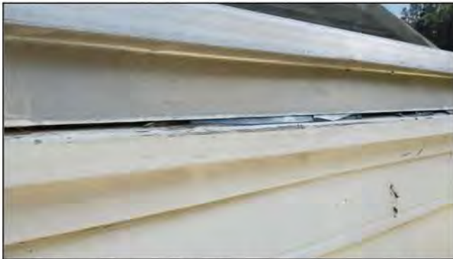
2.4 Item 1(Picture) Broken storm window glass
