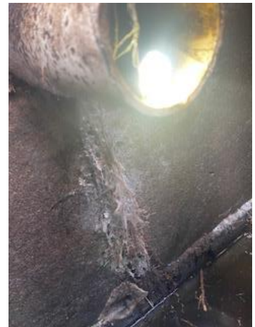
INLET (crack)
