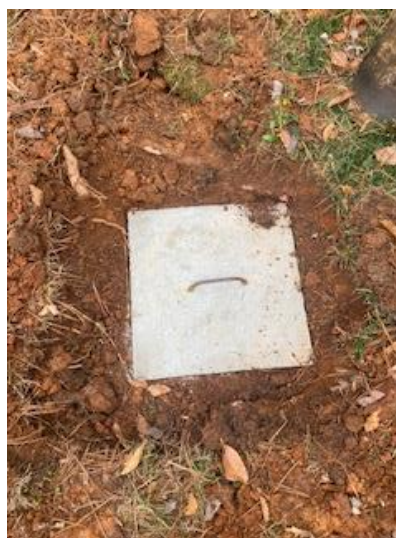
OUTLET lid replaced
