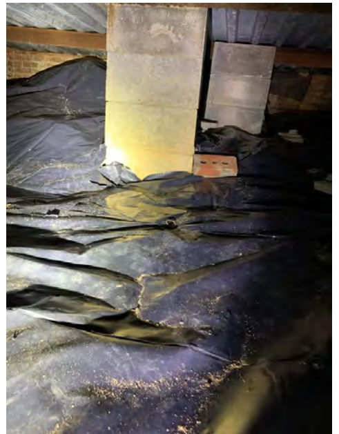
Under front porch
